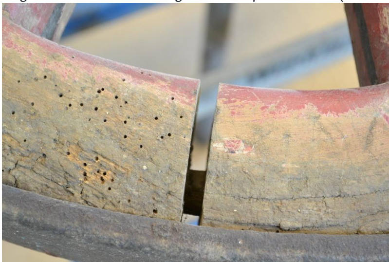
A typical shrinkage gap between felloes of the wheels, also showing old insect damage (MERL 51/1295).
