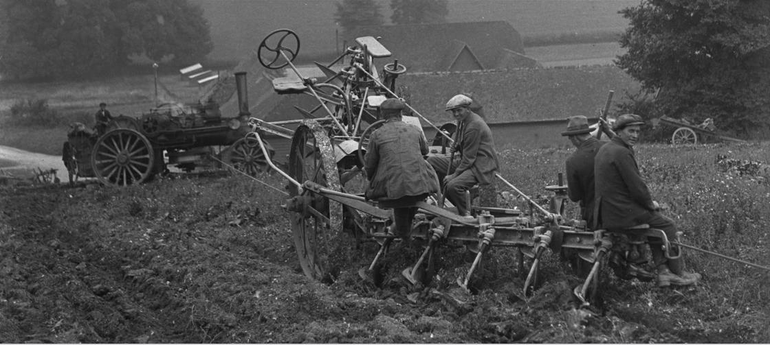
**Key information** John Fowler invented the steam plough. He set up a steam engine at each end of a field. These would then draw a plough across the field by a cable. Usually this was operated by a team who lived and travelled together in a van containing all the equipment.
